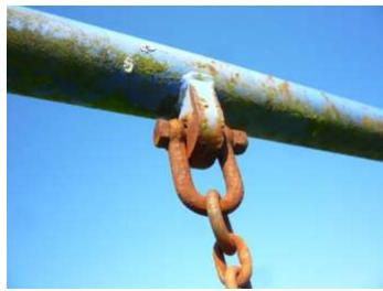
Recommend rub down and remove rust and flaking paint, which has rough and sharp areas - and repaint to prolong life of item - Low risk.
